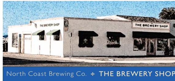
View of Shop from intersection of Pine & Main Streets, looking northwest
